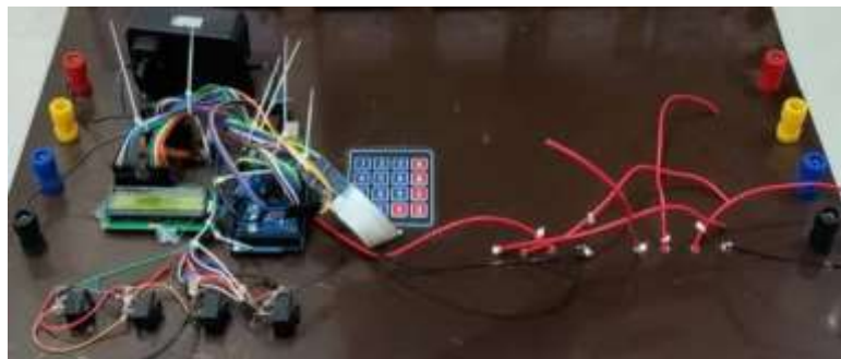
Fig 3: Three Phase Unit
